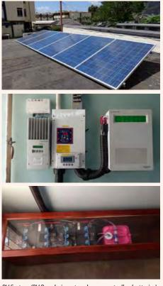
PV System (PV Panels, inverter, charge controller, batteries) used to power PEM electrolyser (September 2014).
